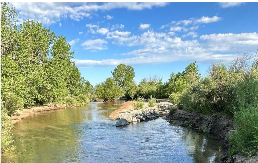
Beginning of beach area- severe erosion behind the boulder edging and of the beach itself, starting a second channel behind the boulder edging
