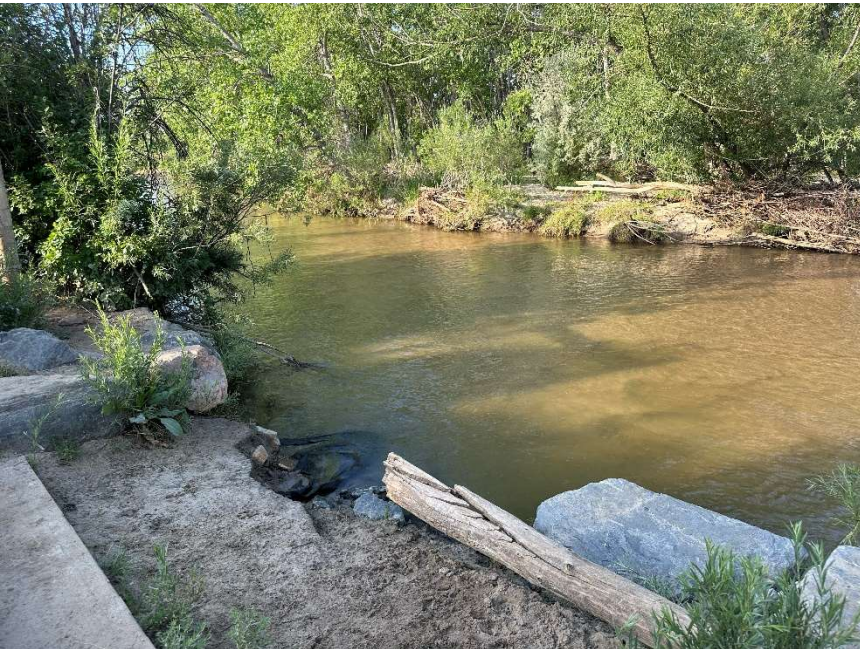
Boulder erosion at Access 6
