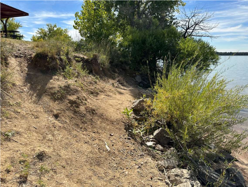
Above flood level bank erosion
